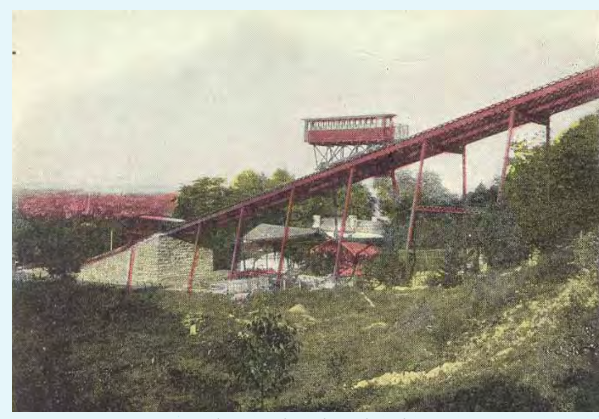
Elevated inclined railway up Escarpment
