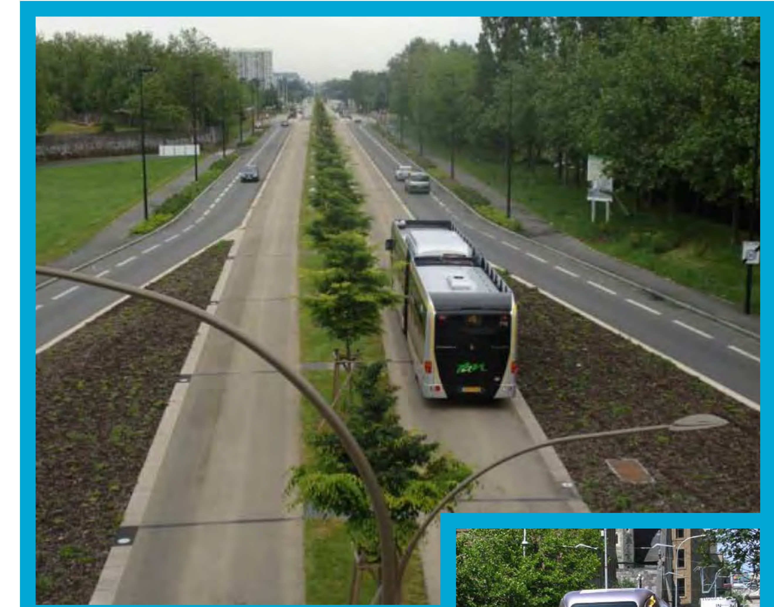
BRT: Nantes, France
