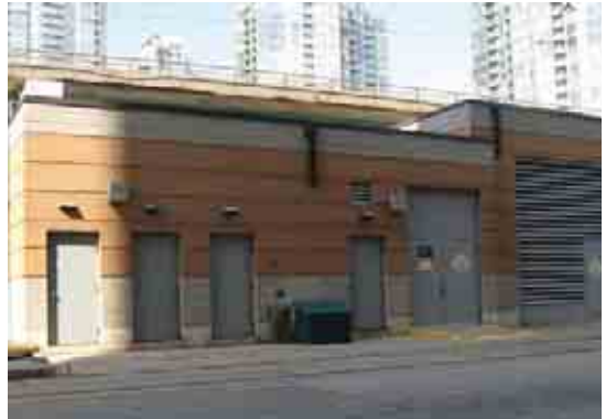
Typical Electrical Substation
