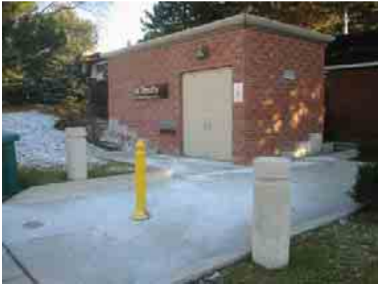
Typical Emergency Exit Building – Sheppard Subway
